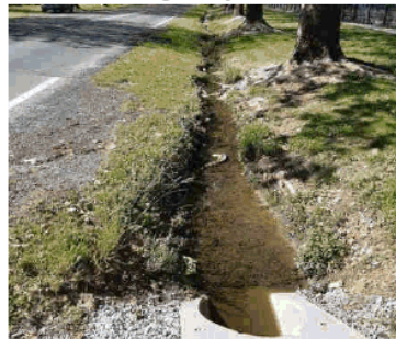
Drainage & trees along eastern side of Park St
