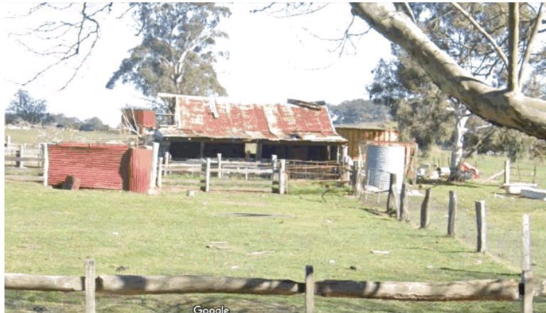
Plate 13: Shearing shed and other outbuildings
