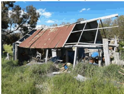
Old Shed western facade
