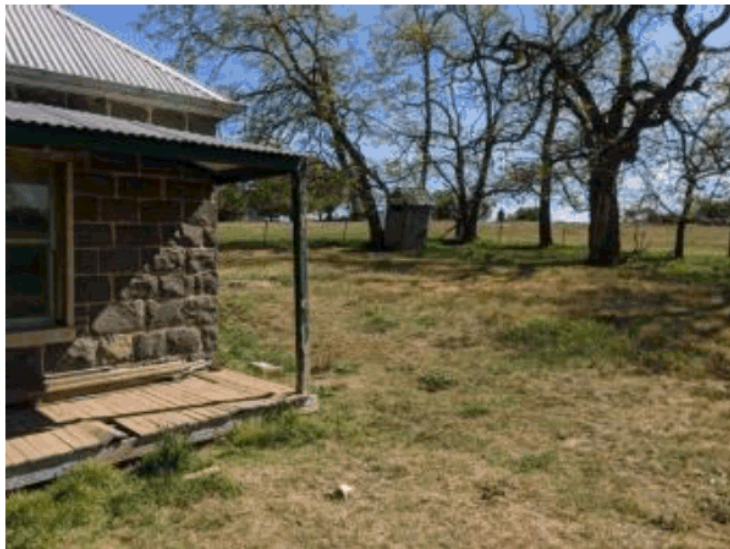
Plate 10: Toilet outbuilding from 2019
