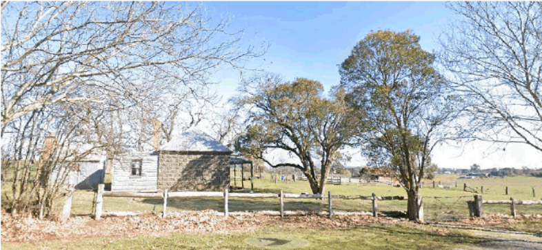
Plate 12: Eastern elevation showing post and rail boundary fence
