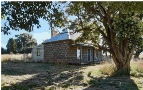
Heritage cottage looking south-west from Park St
