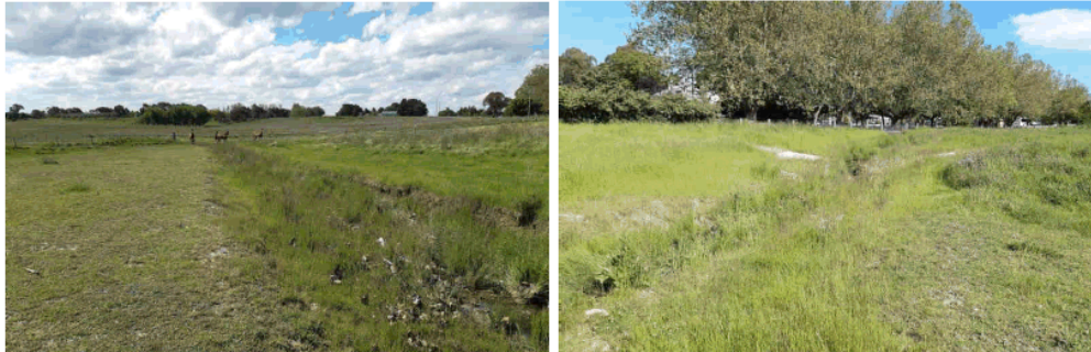
Figure 13: Photos of the Central Watercourse (Drain B) taken November 2021.
