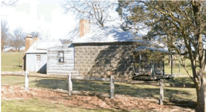
Plate 11: Eastern elevation showing rear kitchen building and skillion addition
